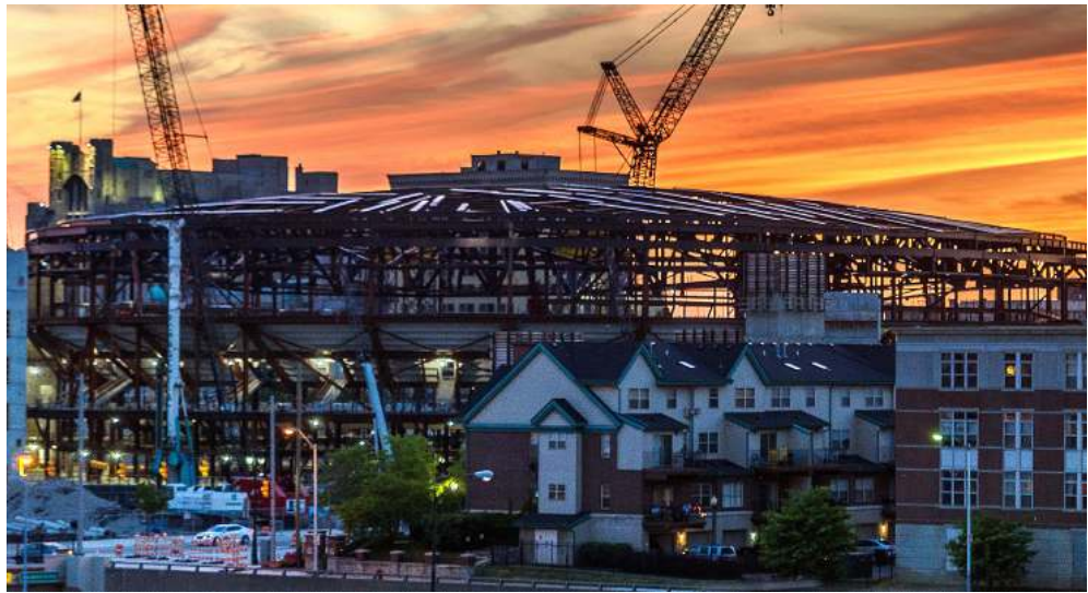
Construction of Detroit's Little Caesar's Arena.
